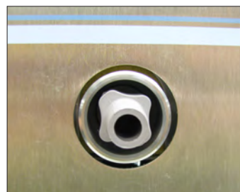
Installed Drain Fitting with Cap Removed
